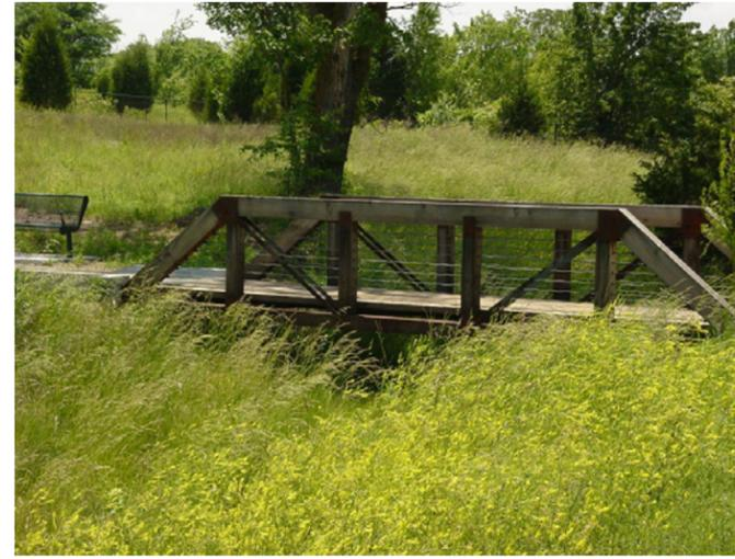
Wood, steel and cable span footbridge
